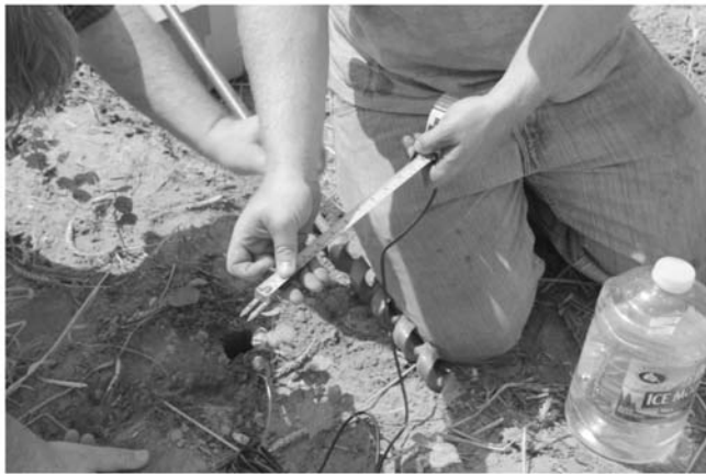
Fig. 4. Getting ready to install an EC-5 volumetric moisture sensor.
